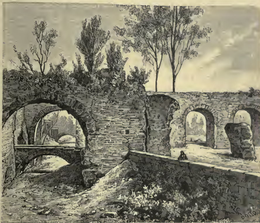
Naples—Arcade of the Aqueduct called Ponti Rossi.
